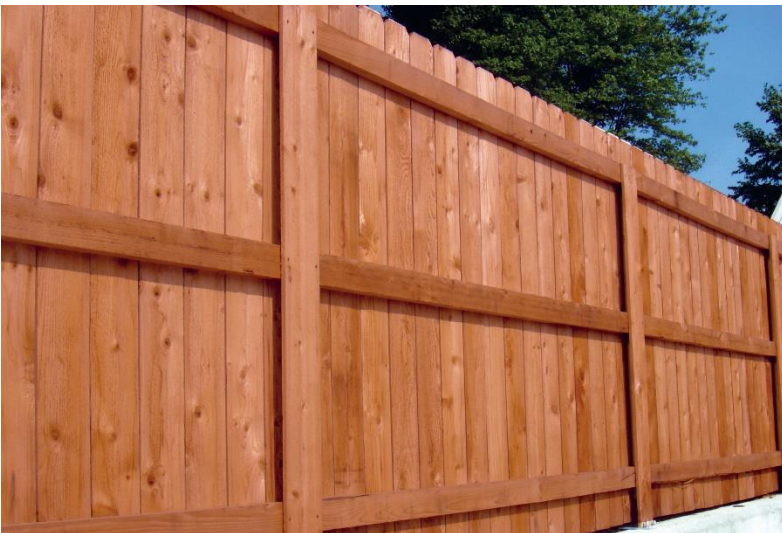
Three-rail style for the yard side of the fence using steel posts hidden by beauty boards. Picture frame fence will have horizontal cap board on top of fence, not open board tops as shown in this photo. (Disregard the stain color in the photo.)
